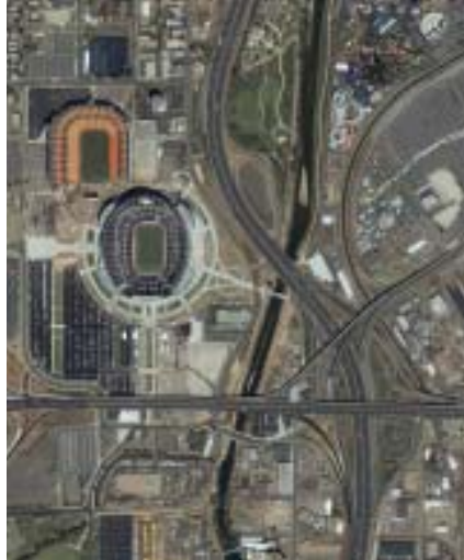
More than the sum of its parts: complex systems, such as highways, are constantly evolving.
